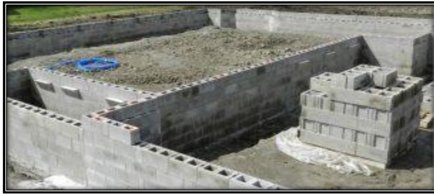
(fig.25 Pre-cast Foundation Technique)
