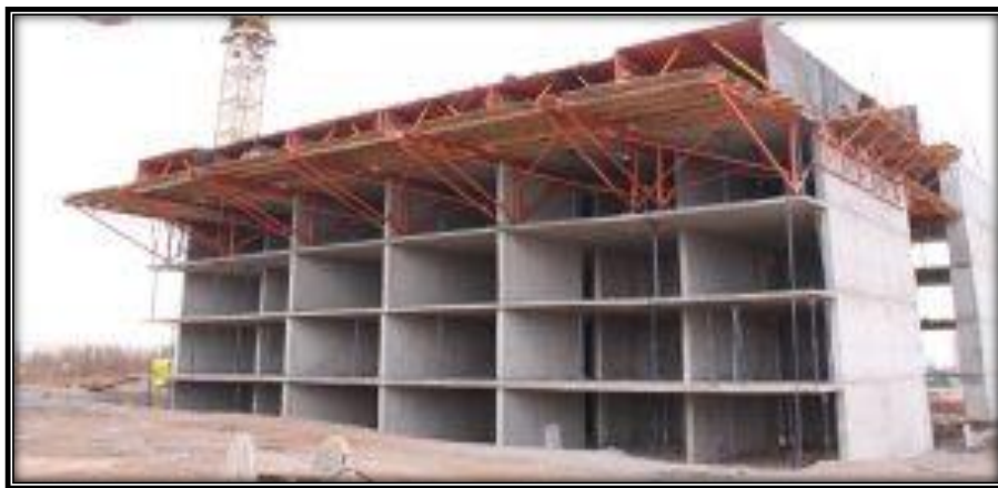
(fig.24 Tunnel Formwork System)
