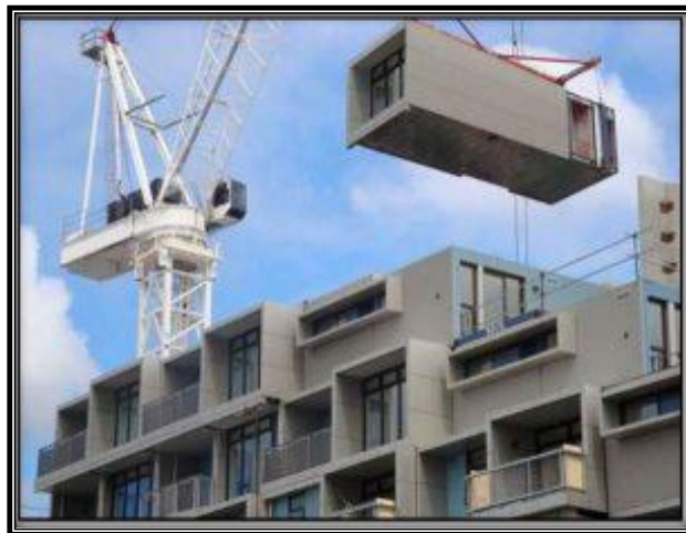
(fig.22 3D Volumetric Construction)
