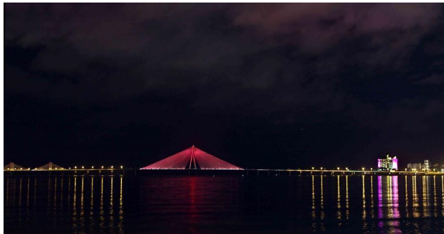
(Fig no.11 bandra worali se link bridge)
