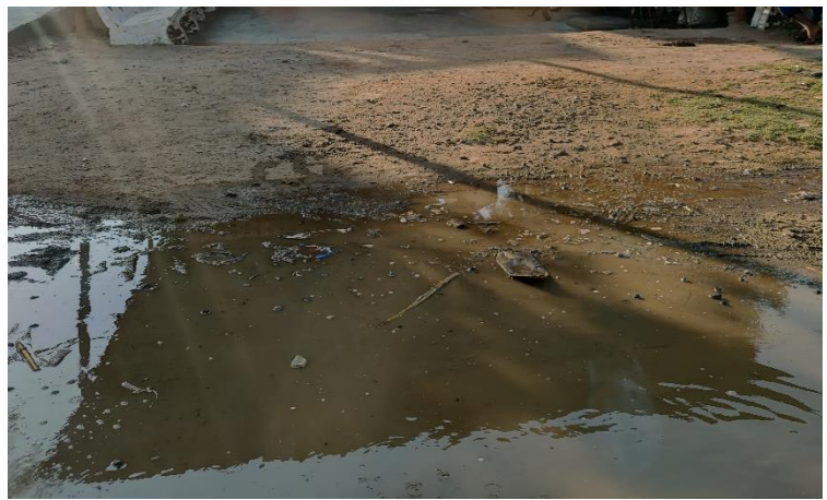
(Fig no.16 existing condition in valasan)
