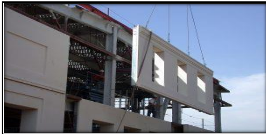
(fig.26 Hybrid Concrete Building Technique)
