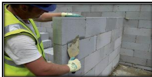
(fig.27 Thin Joint Masonry Technique)
