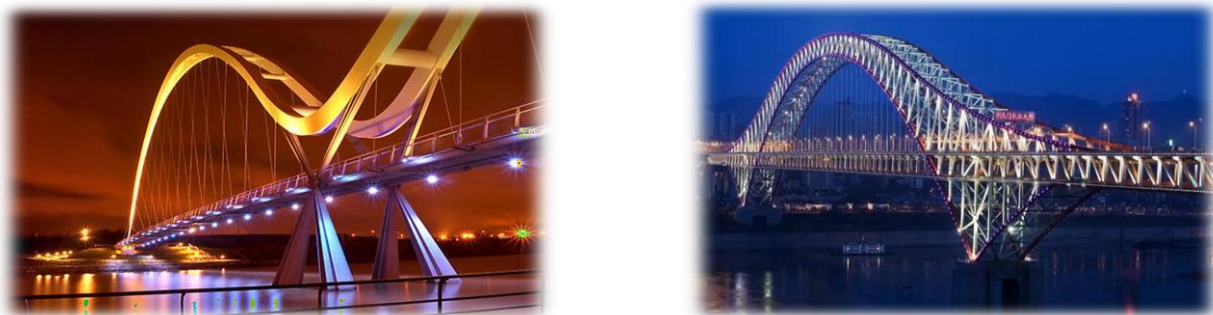
(Fig no.10 bow string bridge)
