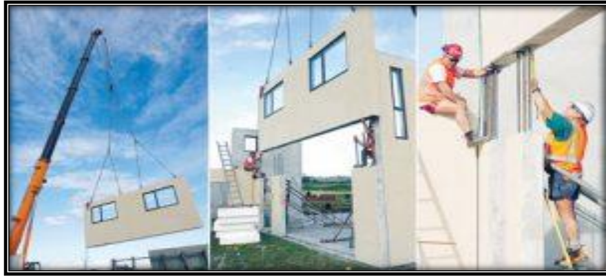
(fig.23 Precast Flat Panel Modules)
